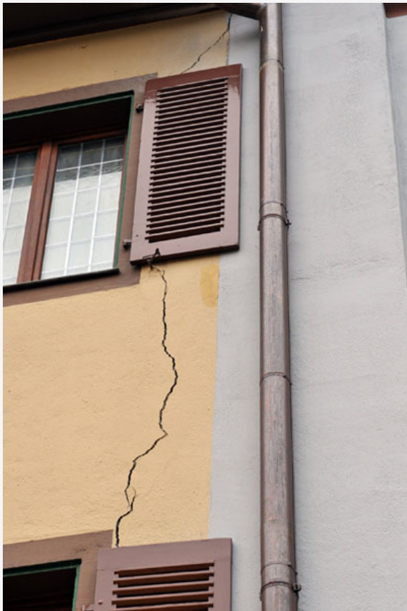
e.g. Staufen in Germany (transition of anhydrite to gypsum)
