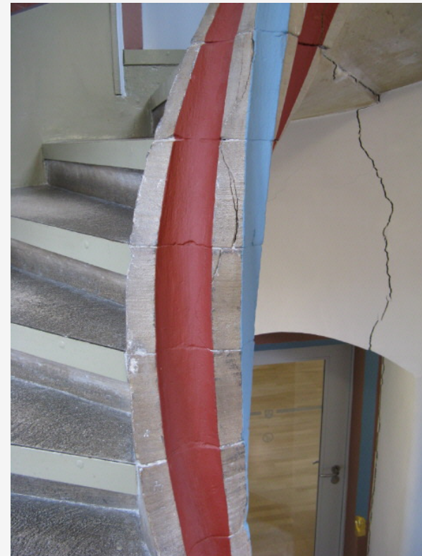
e.g. Staufen in Germany (transition of anhydrite to gypsum)
